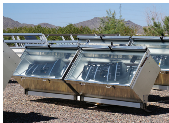
Type F2 (Arizona) - fixed elevation, tracking azimuth
